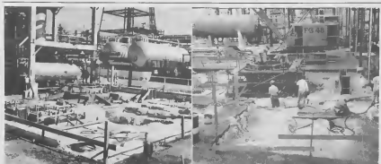
FOUNDATIONS are prepared at AAR-I and NFAR. FUNDISHAN TA wordé prepará na AAR-I y pa instalacion di two towers, one to debutanize NFAR pa instalacion di dos tower, uno pa debutanizá y otro pa deparaffinazá gasolin.
